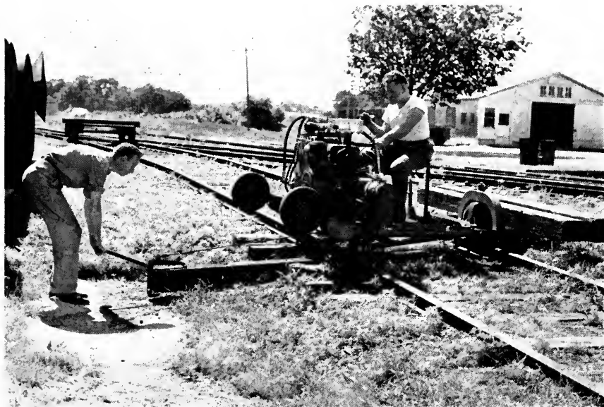
Hydraulic tie inserter.
